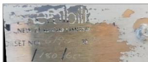
The fire door set is a system, and the frame and doors must be installed in accordance with the specifications before the tags stating the fire rating can be applied. Please ensure that the tags for new doors are installed promptly. Take care not to damage or paint over the tags.
